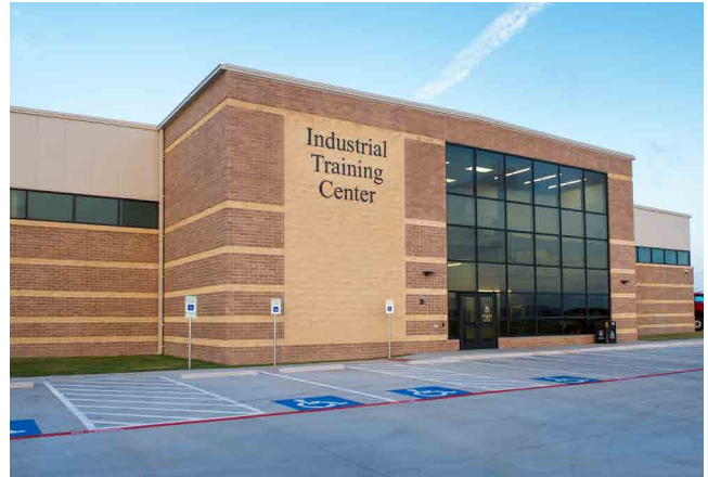
VC EMERGING TECHNOLOGY COMPLEX INDUSTRIAL TRAINING CENTER 7403 Lone Tree Road, Victoria, TX 77905
