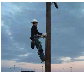
Power Line Worker + $37,000-$69,000 12 Weeks: per level, 3 levels
