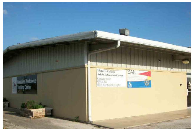
VICTORIA COLLEGE GONZALES WORKFORCE TRAINING BUILDING 1828 Saint Paul Street, Gonzales, TX 78629
